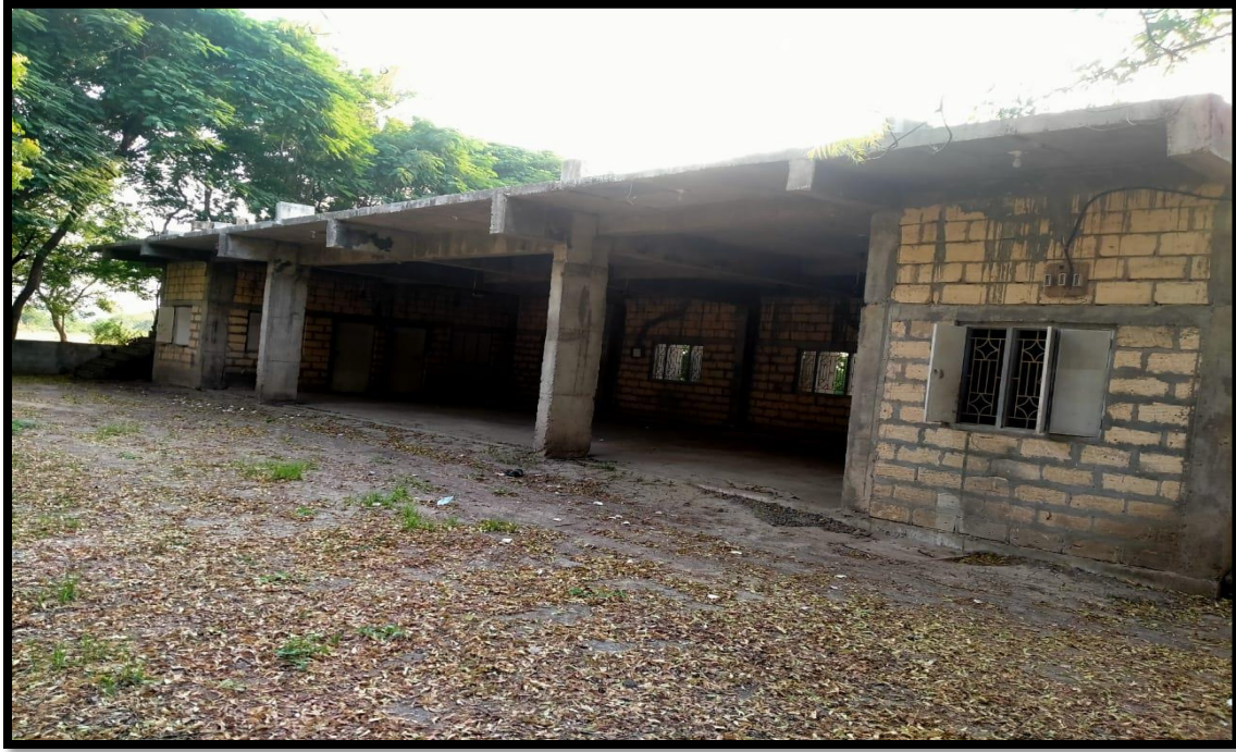
(figure 4.17 Community Hall in Katawana )
