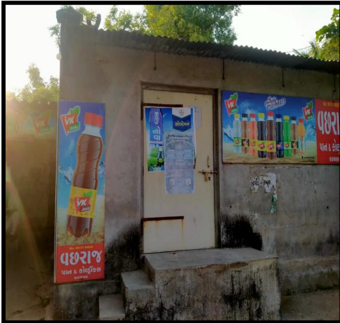
(figure 4.15.Panchayat Building in Katawana )
